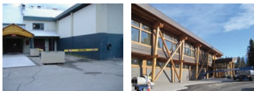
Rec Centre before and after reconstruction
