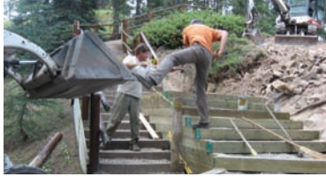
Building new staircase on Bow Falls Trail
