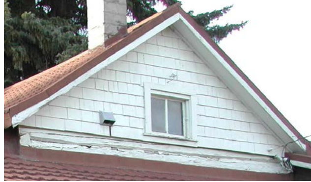
Photo 8 – Gable end detail
