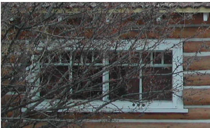
Photo 11 – North façade window detail
