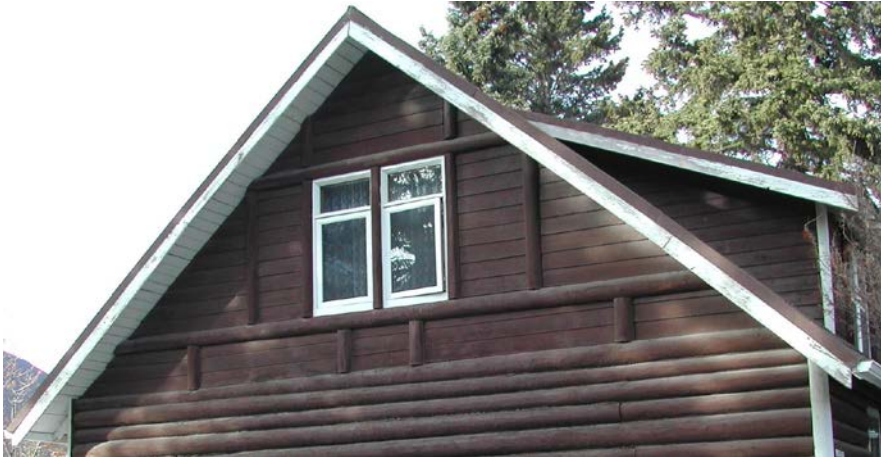
Photo 7 – Gable end detail
