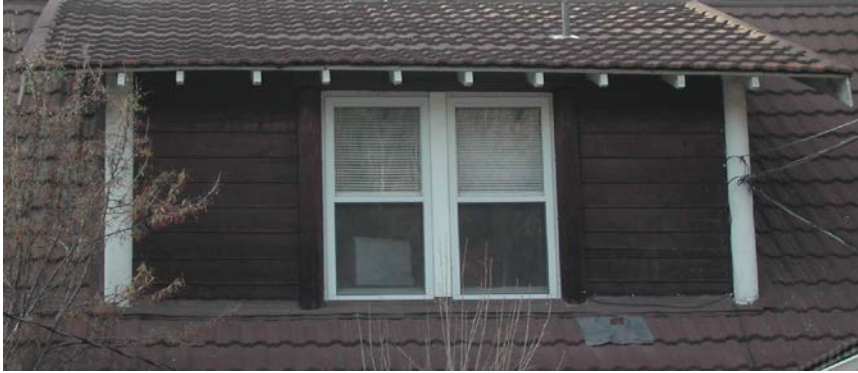
Photo 9 – Shed dormer detail
