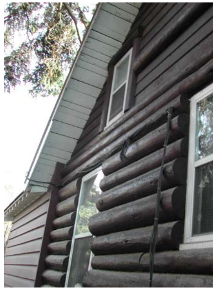
Photo 11 – North façade window detail
