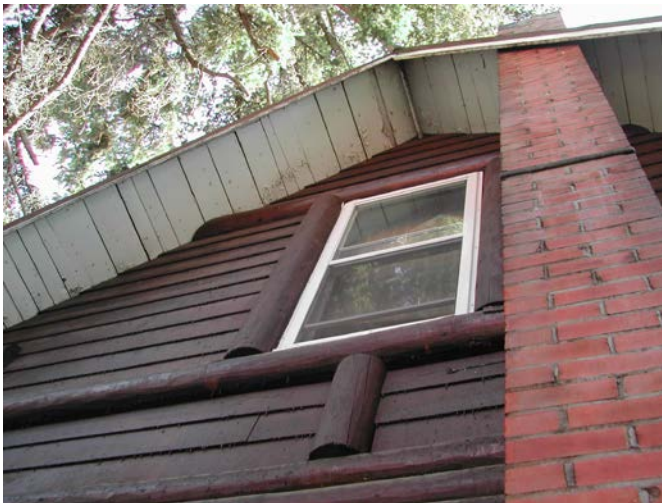
Photo 12 – Gable end detail
