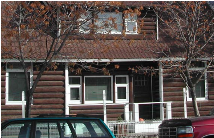
Photo 2 – Inset porch and window detail
