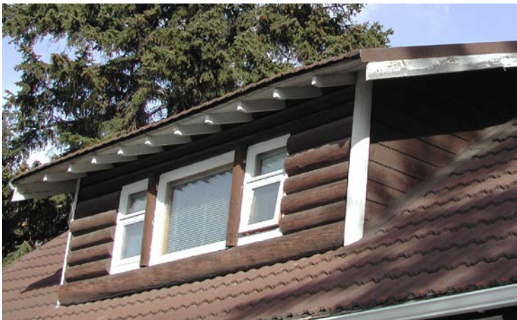
Photo 4 – Shed dormer detail
