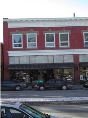
Photo 7 – 103 Banff Avenue storefront
