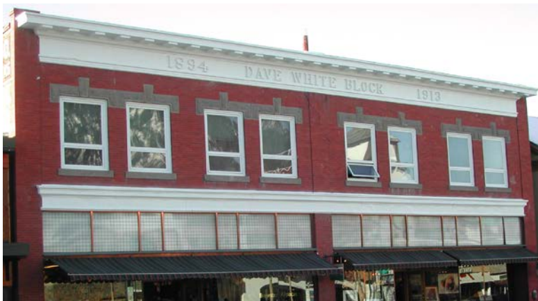
Photo 6 – second storey, beltcourse, clerestory and awning detail
