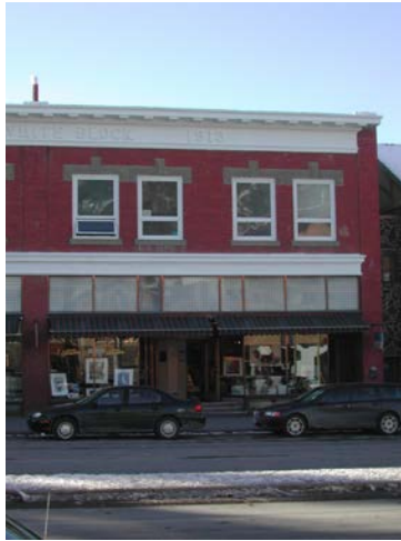
Photo 8 – 105 Banff Avenue storefront
