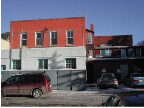
Photo 26 – West (rear) façade
