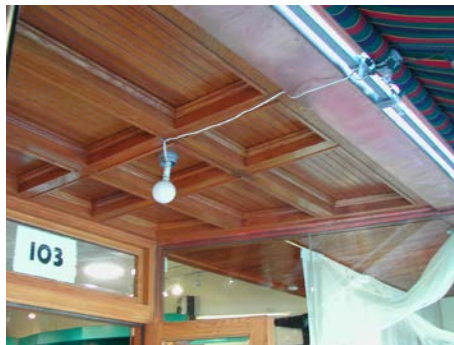
Photo 12 – 103 Banff Avenue storefront
