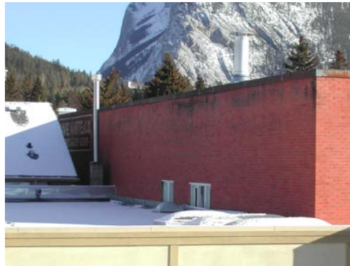
Photo 23 - North façade from lane
