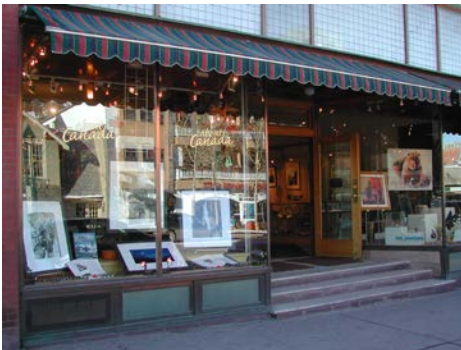
Photo 17 – 105 Banff Avenue storefront
