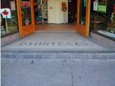
Photo 13 – 103 Banff Avenue storefront
