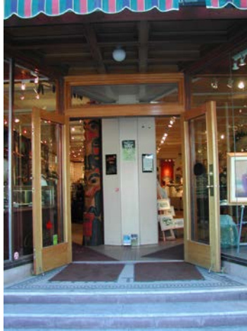
Photo 14 – 105 Banff Avenue storefront
