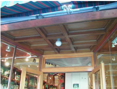
Photo 15 – 105 Banff Avenue storefront
