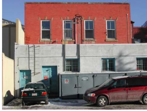
Photo 27 – 105 Banff Avenue - west façade
