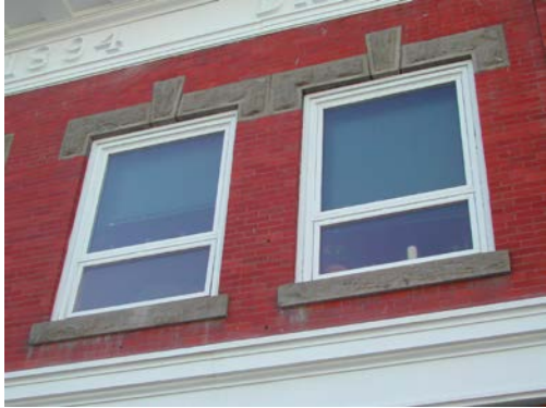
Photo 2 – second storey window detail
