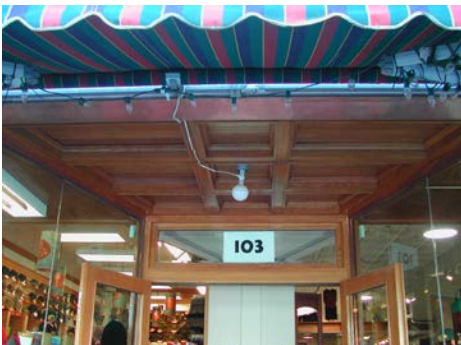
Photo 11 – 103 Banff Avenue storefront
