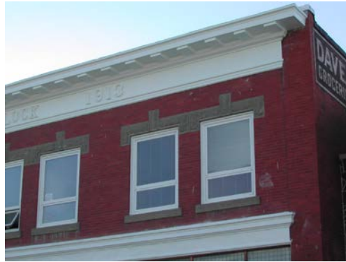
Photo 3 – second storey window detail
