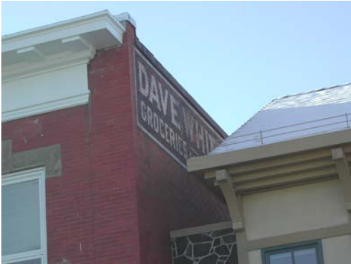
Photo 22 - North façade from Banff Avenue
