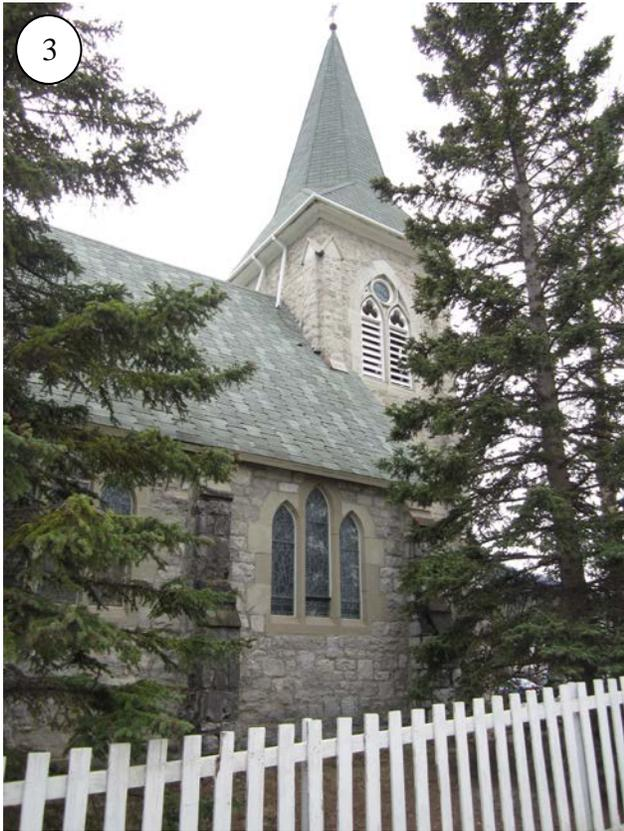
Photo 3: North and east sides of bell tower (depicting stonework, roof form sandstone tracery around stained glass windows and bell chamber)
