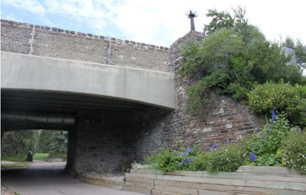
Rundlestone Retaining Wall – North
