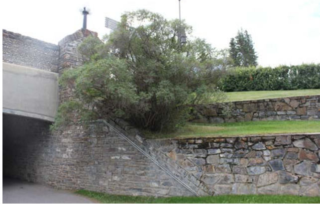
Rundlestone Retaining Walls – South
