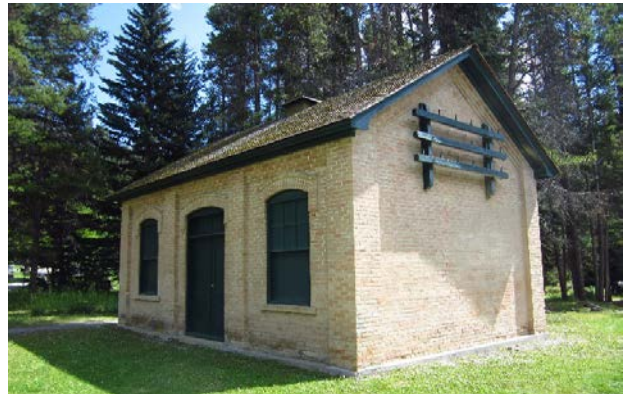
Eighteen (18) Wood Insulators over Three Wooden Planks supported by Two Wooden Brackets
