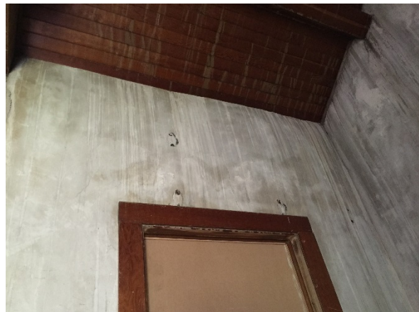
Open Gable Ceiling with Exposed Wood Paneling,
